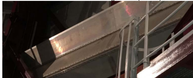
Clay Observatory Windscreen: Continuous Piano Hinges
