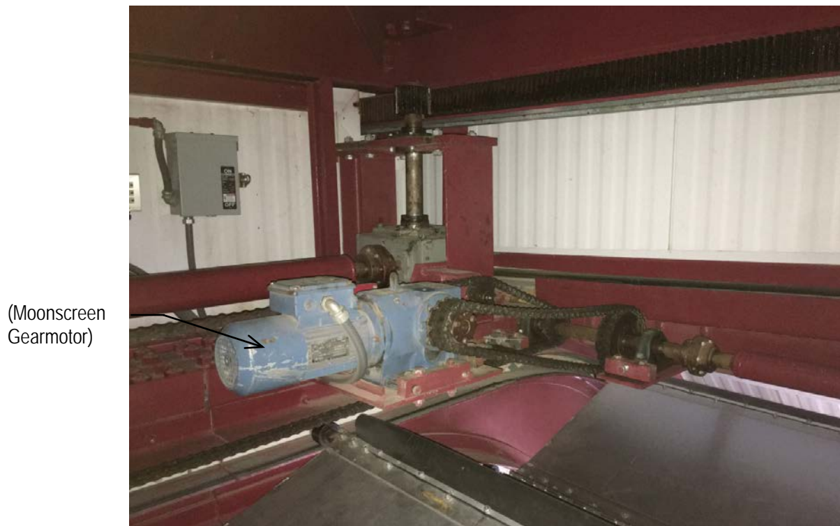
Upper Shutter Drive – TSPM (above) and Magellan (below)
