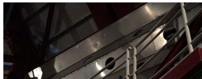
Baade Observatory Windscreen: Intermittent Piano Hinges
