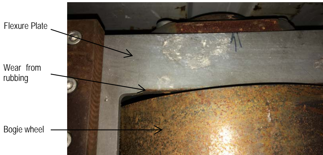
Magellan Flexure Plate Wear from Wheel/Axle Slippage
