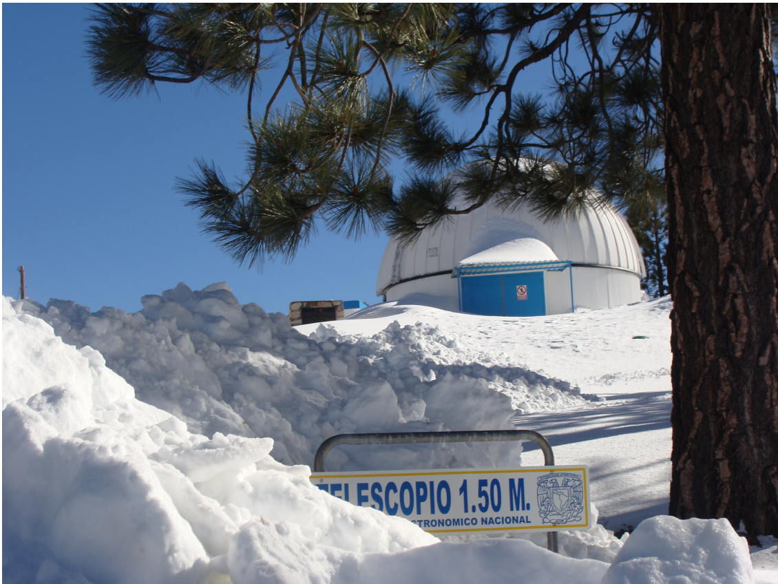
Figure 19: This photo shows the dome for the 1.5m telescope as access was restored to the OAN-SPM after the severe winter storm in January 2010. Photo courtesy of Ignacio González.
